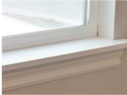
3 WAY DRYWALL WINDOW WRAP, PAINTED POPLAR SILL AND APRON (PROFILE OF YOUR CHOICE)
