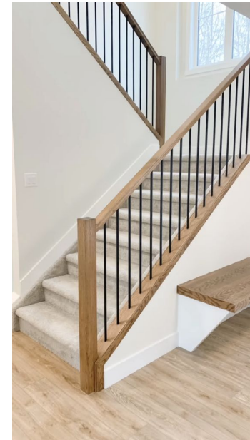
STAIR RAIL OPTION 2 WOOD RAIL AND NEWEL POST WITH PAINTED OR IRON BALUSTER
